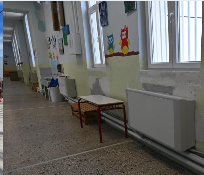
Fan coils inside the school building of Evros.
