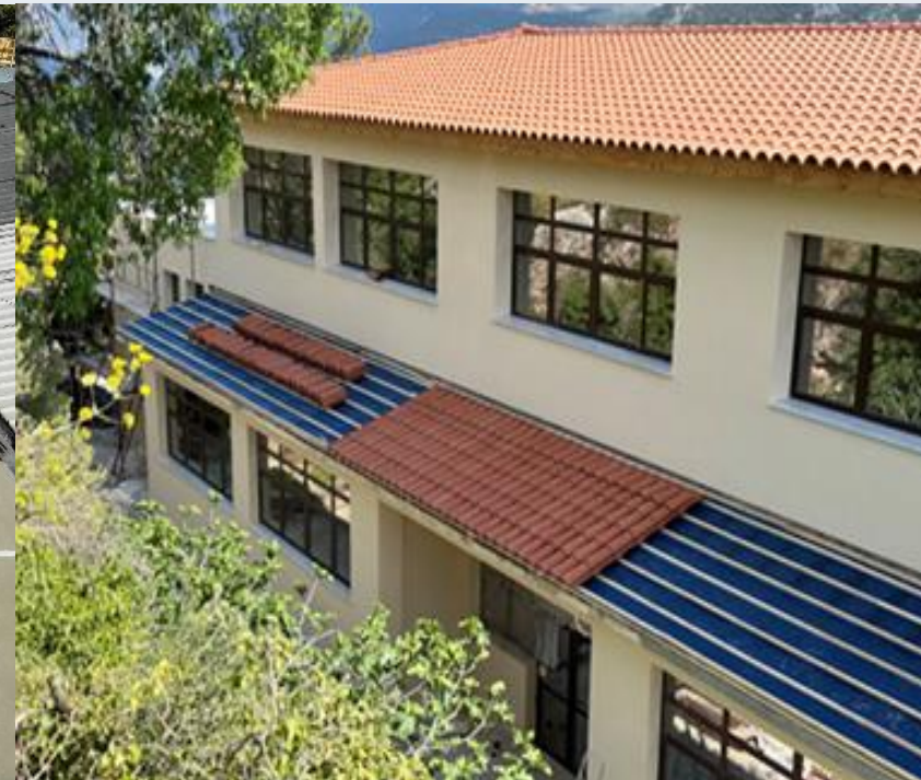
Thermal insulation on the tile roof of the Delphi Art Station of the Athens School of Fine Arts.
